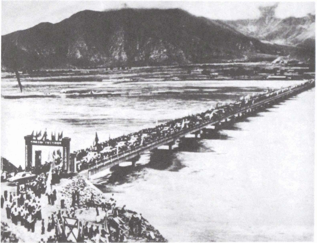
Chushul Bridge, the largest on the Yalutsangpo, links Lhasa with Laka Shigatse and other areas.
